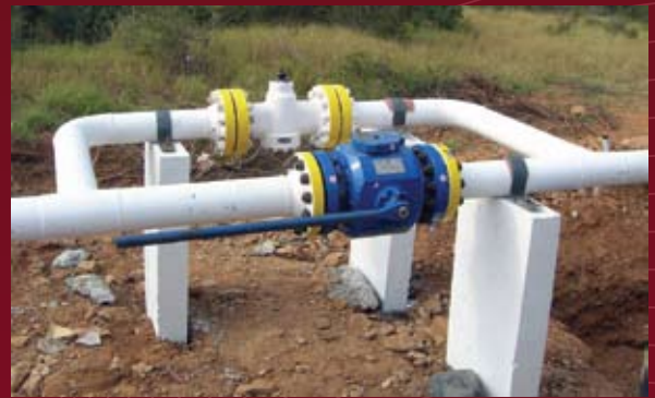
6" 600 ANSI Receiving valve, with full 6 inch bypass.
